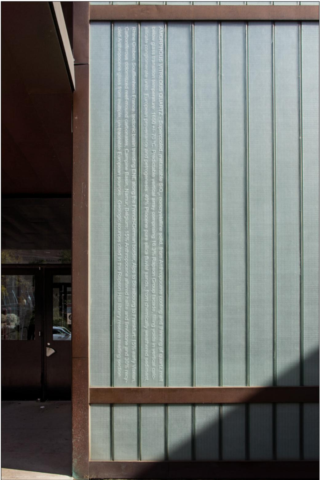
Fig. 143. Rapson Group (Geology Text Panels) / Glass, west wing, Holl annex, Rapson Hall, approximately, 11 ft. x 16 in. etched, Proflit glass.
